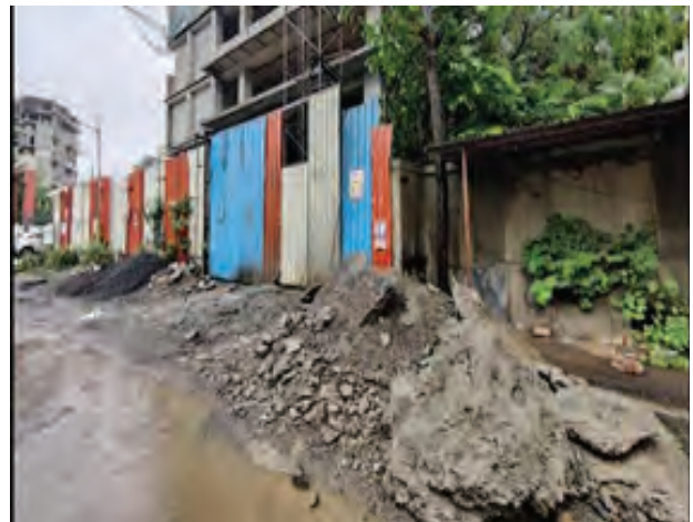
Fig. 4: Dumping of C&D waste illegally done outside the construction premises of Pune City
