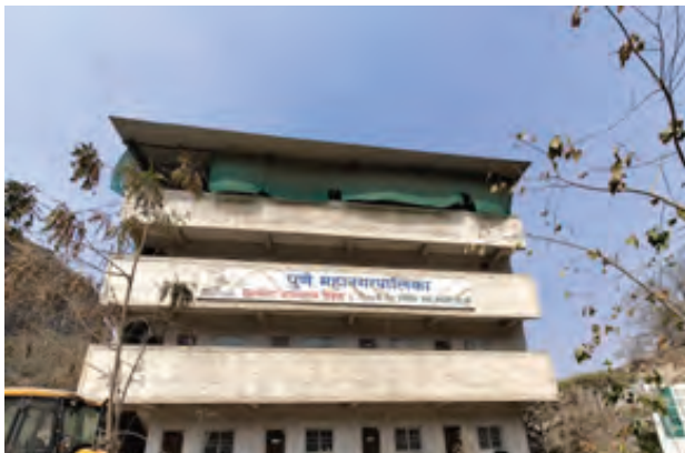
Fig. 6: C&D waste processing plant at Wagholi
