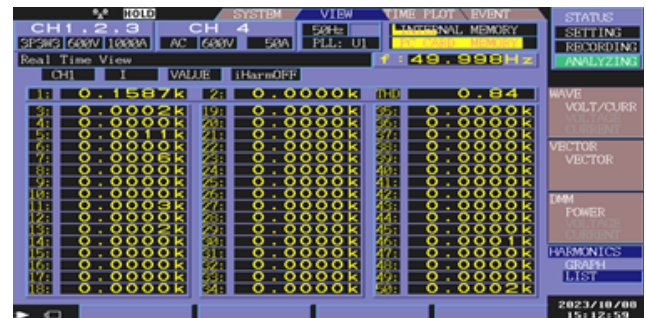
Figure 6: VFD output voltage harmonic measurement at full load
