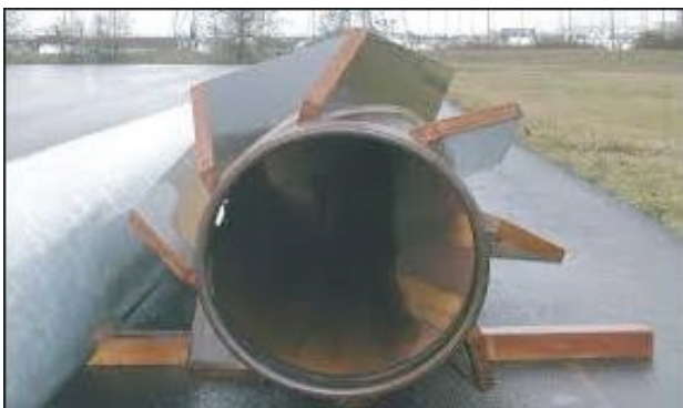
Fig. 2: Cross-section view of spin fin pile
